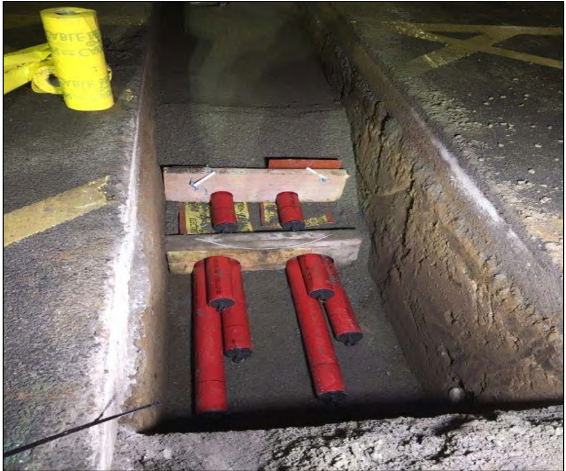
Plate 2.1 Typical Trench Views
