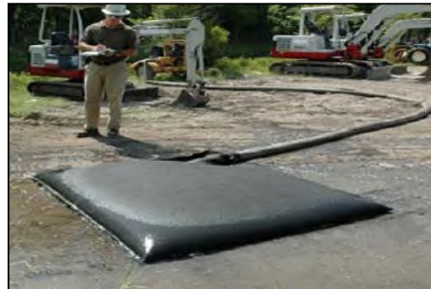
Plate 4.2 Silt Bag under inspection
