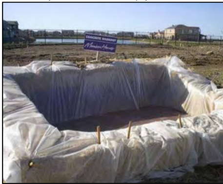
Plate 3.1 Concrete washout area
