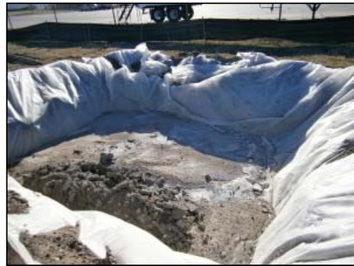
Plate 3.2 Concrete washout area
