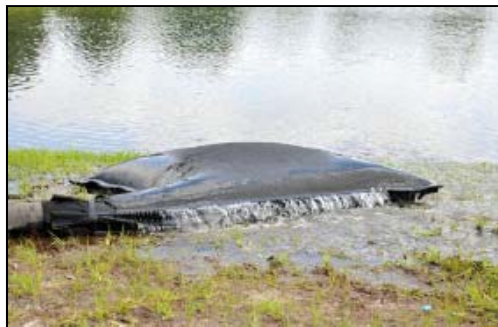
Plate 4.1 Silt Bag with water being pumped through
